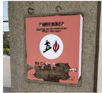
8. Parking Structure Pedestrian Signage ●
